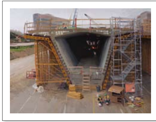
08-032 Casting a Segment
