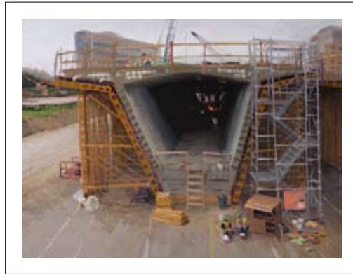
08-032 Casting a Segment
