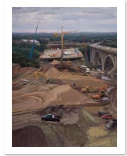
08-028 Piles of Dirt: The Bridge Site from the West Bank
